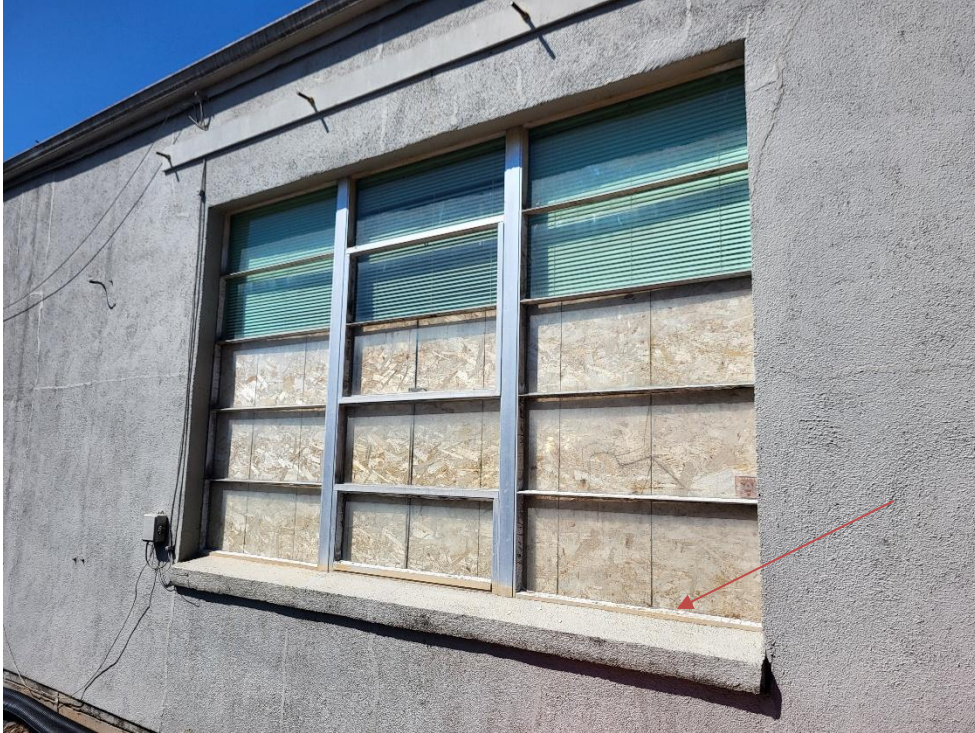
Photo 9 – Wood Shop: Window Glazing = 2% Chrysotile Asbestos
