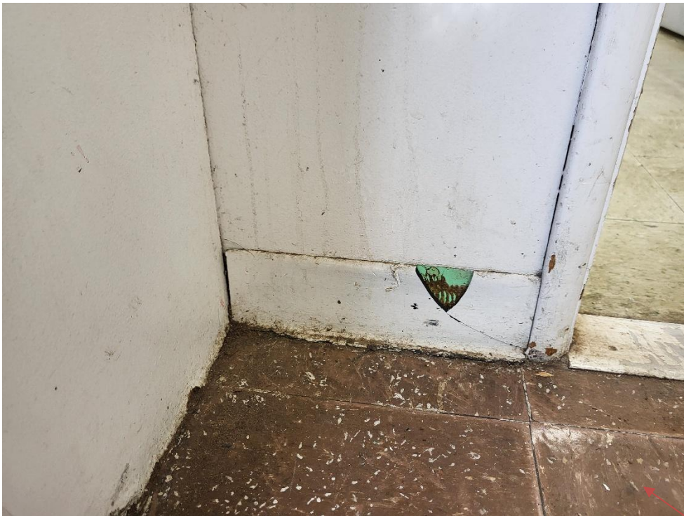
Photo 10 – D4: Red Vinyl Floor Tiles = 3% Chrysotile Asbestos
